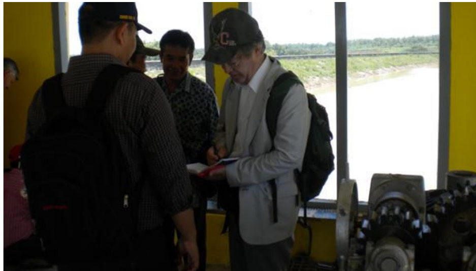
Gate operation Room
