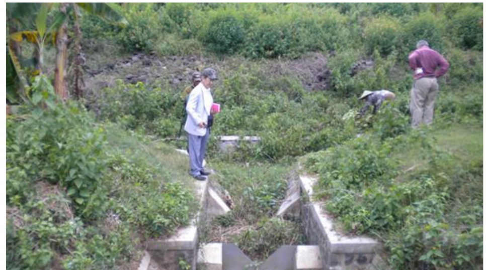
Seepage Monitoring Weir
