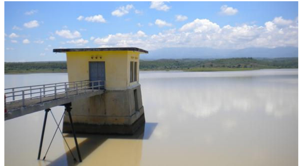
Intake Tower of Dawuhan dam
