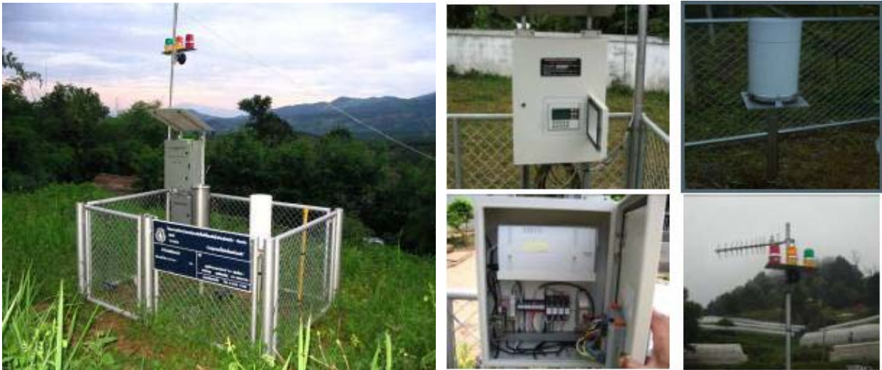
Figure 6.1 - 1. Automatic Early Warning System
