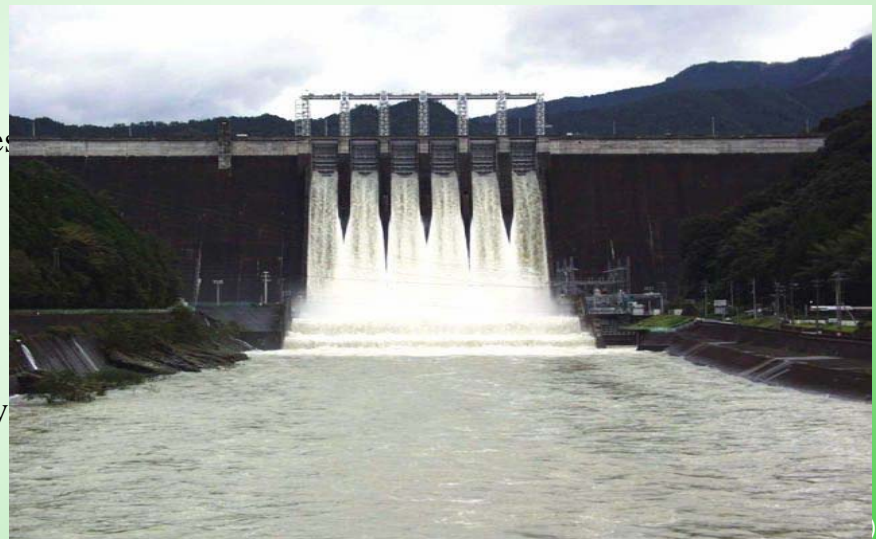
Discharging from spillway at Sameura Dam
