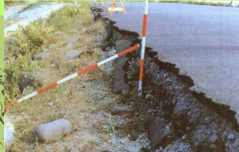
Crest of Makio Dam was damaged by the earthquake.
