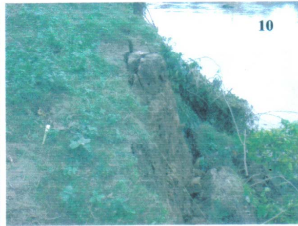
Photoes (7 to 10) showing earth slide and soil condition of breach portion of embankment
