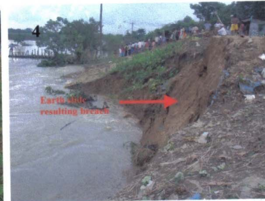
Photoes (3 to 4) describing a reason for breach at Bara Alampur, Devidwar, Comilla
