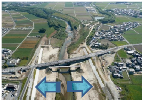
River widening, Excavation
