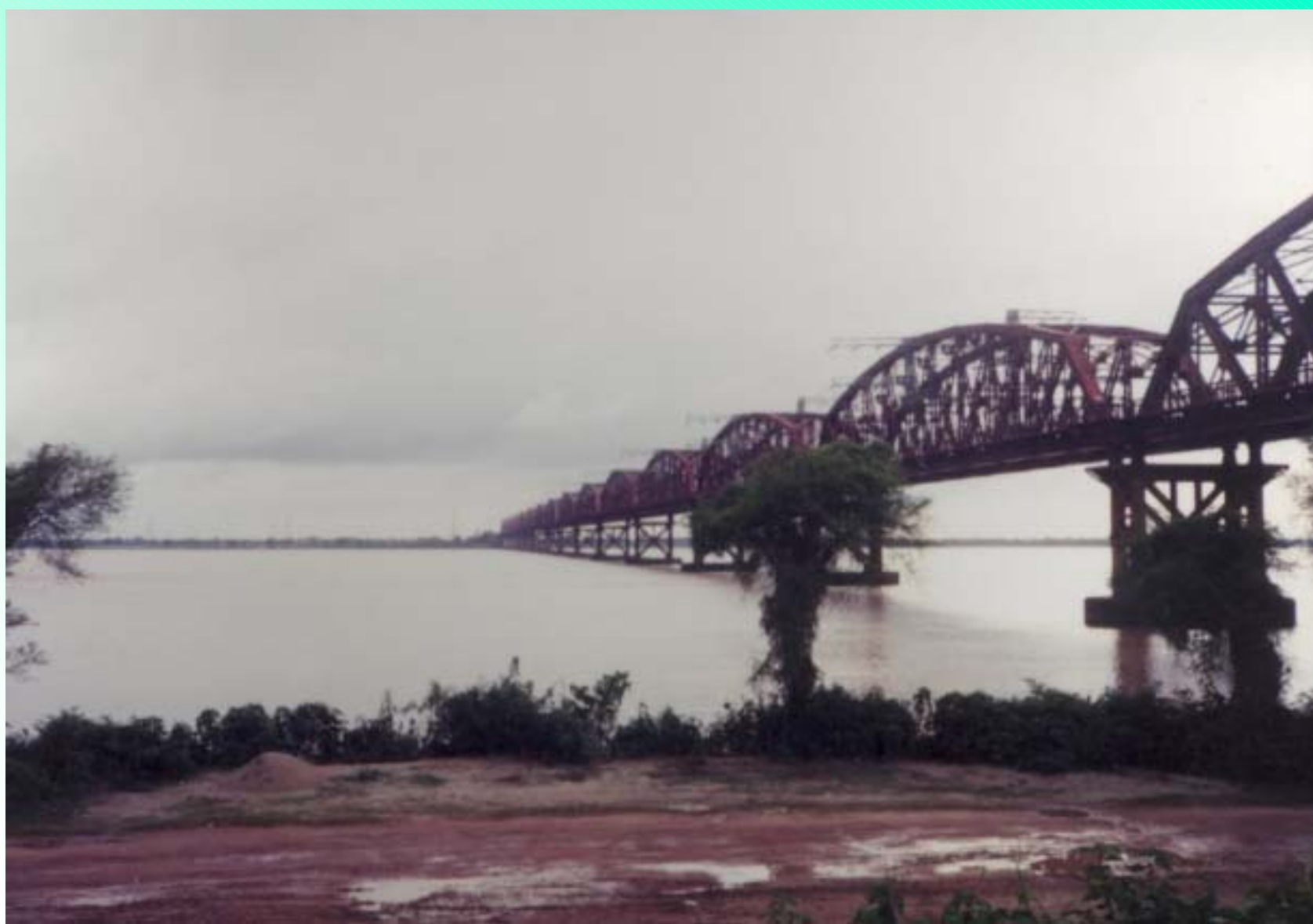
GANGES AT HARDINGE BRIDGE (During monsoon)
