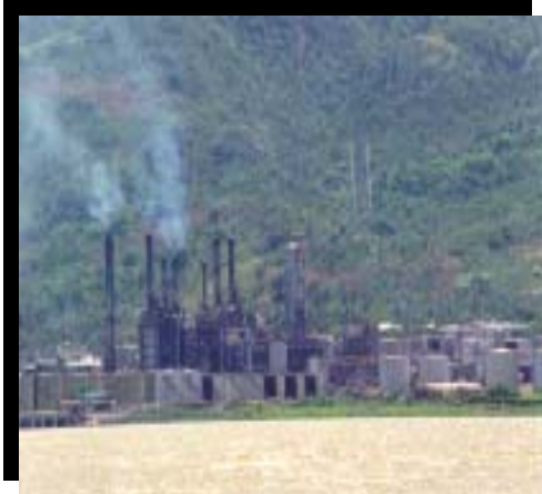
Industrial cooling water
