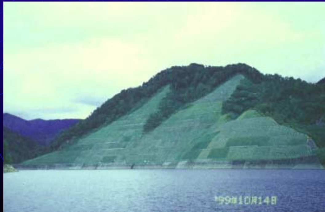
Revegetation on Excavated Slopes
