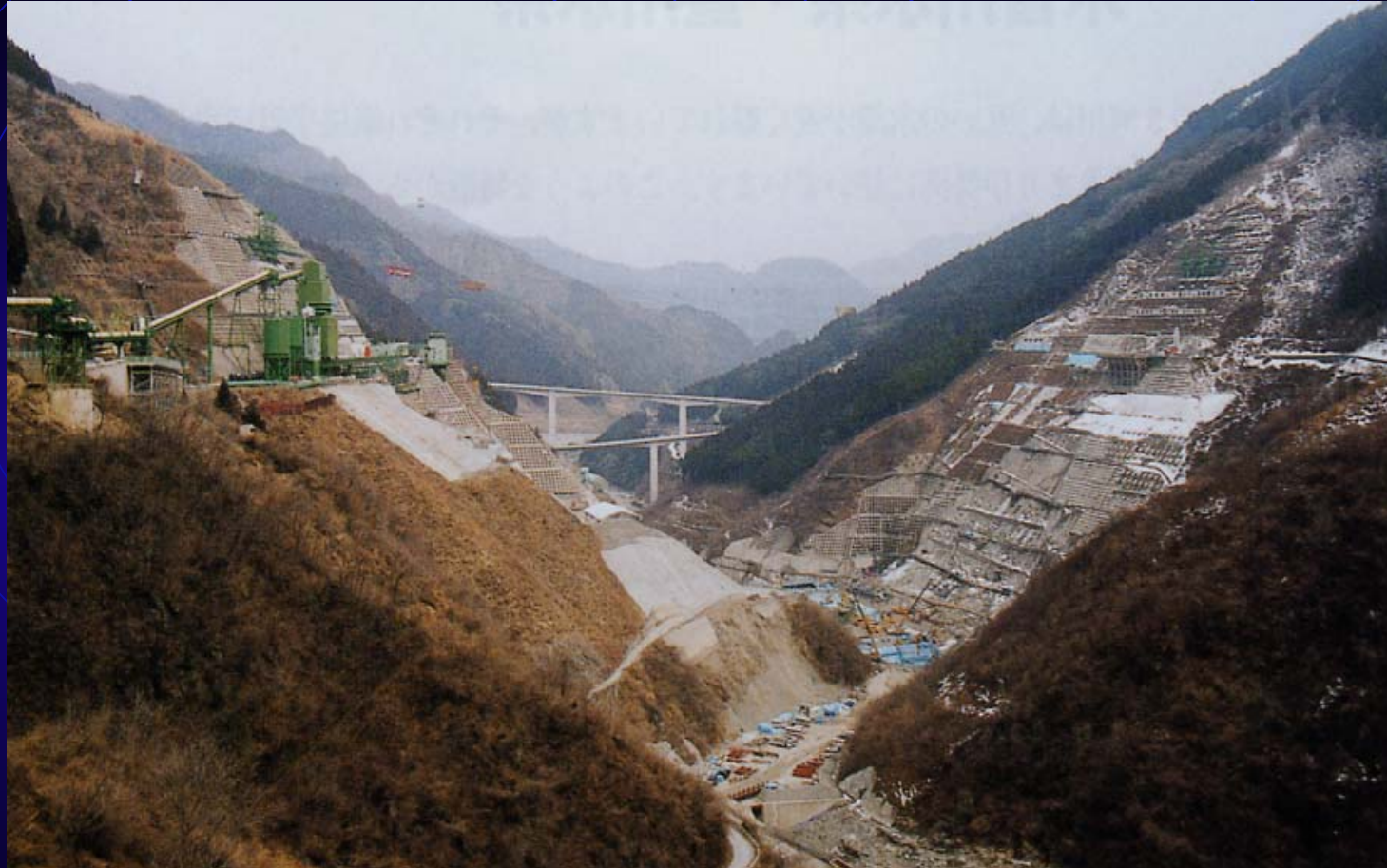
Takizawa Dam (Under Construction)
