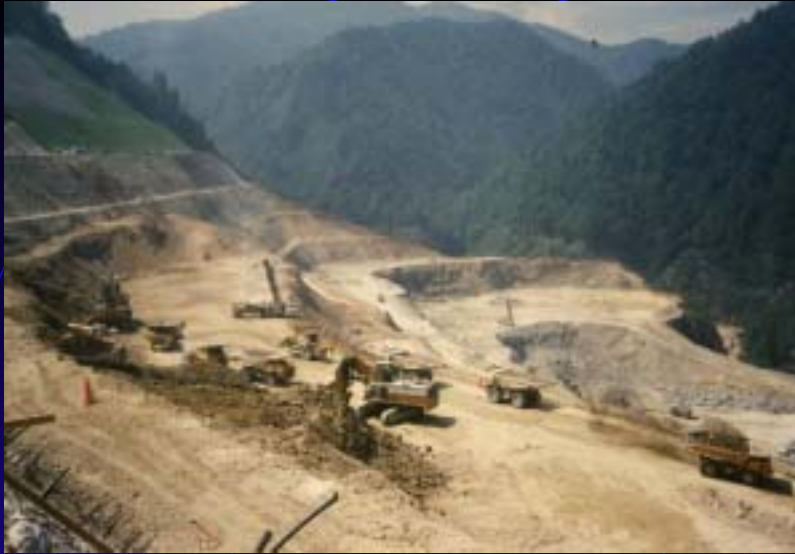
Quarry Site for Rock Material
