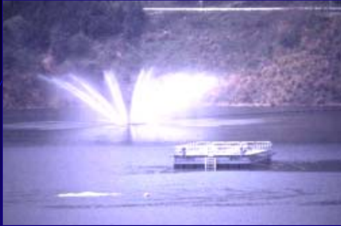
Hypolimnion Aeration (front) and Surface Aeration (back)
