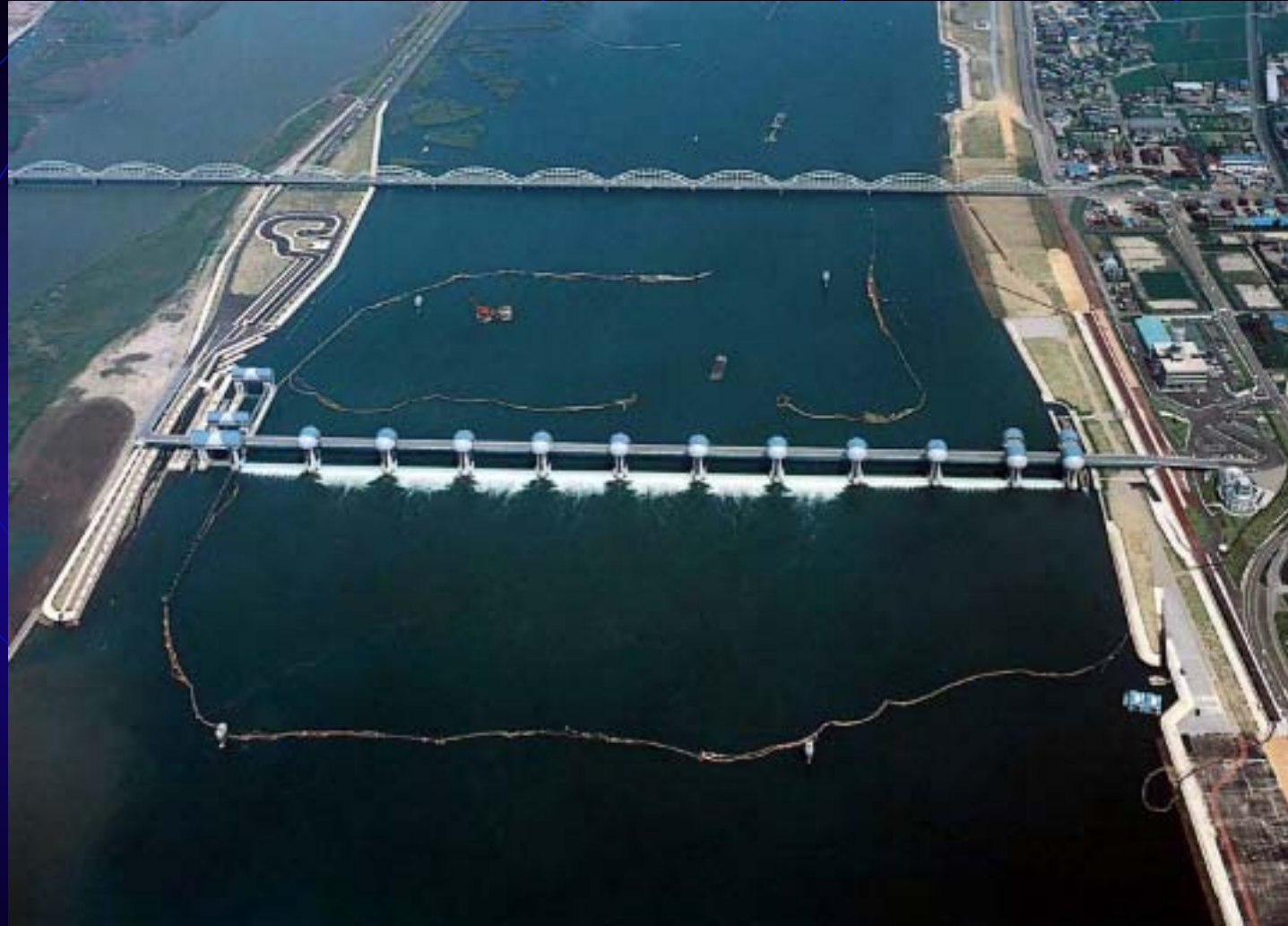
Nagaragawa Estuary Weir
