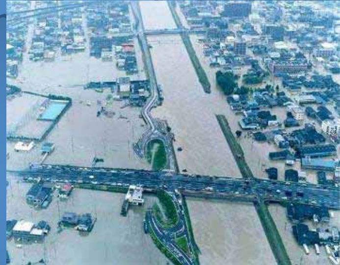
Flood in Tokai Area (Sep. 2000)
