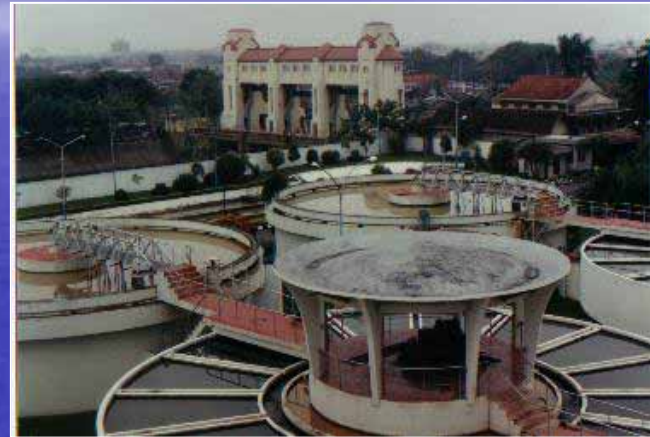
Water Supply (PDAM)
