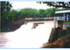
Jati Rubber Dam
