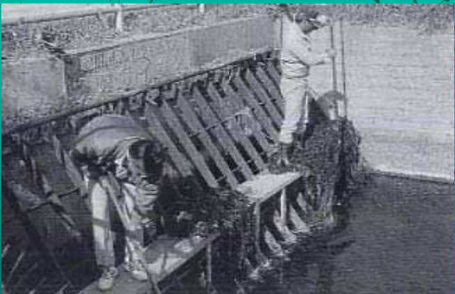
Removing litter of main canal
