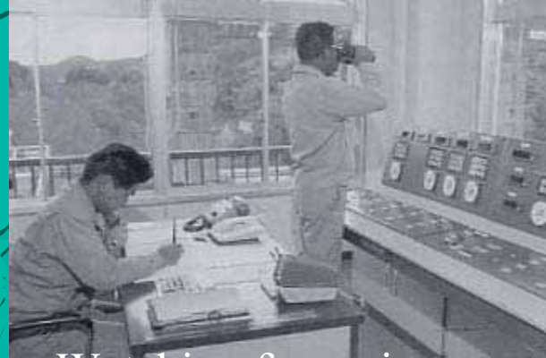
Watching for main facilities and operating
