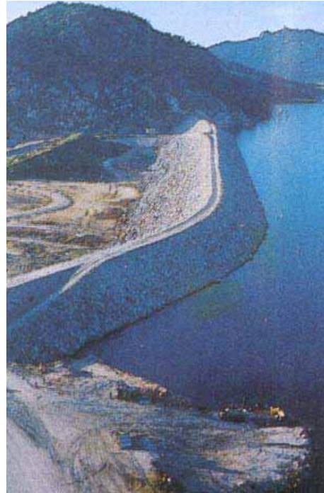
Maduru Oya Dam
