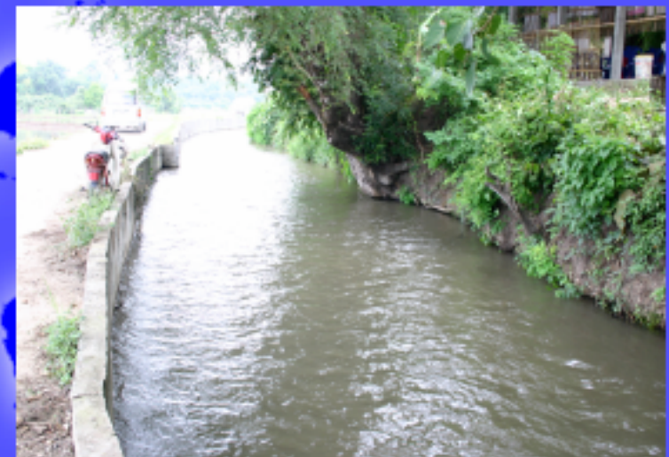
Canal construction almost founded by farmers' irrigation association (Chiang Mai)
