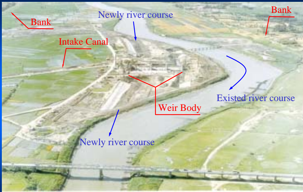
Akigase Diversion Weir in construction (photographed in 1964 (Jpn))
