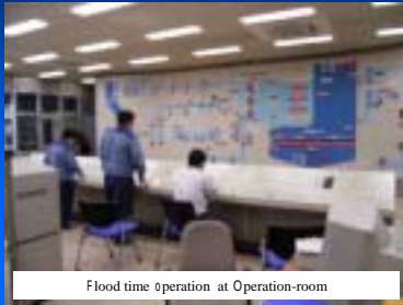
Flood time operation at Operation-room
