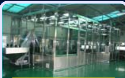
Water Bottle Plant Inner-view
