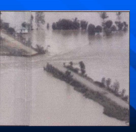
Collapse of embankment of national road No 1 by overland flow from right bank side of Mekong River during the flood in year 2000
