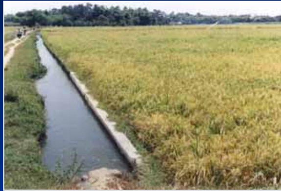
Irrigation Area = 304,000 ha (121,000 ha from reservoirs)
