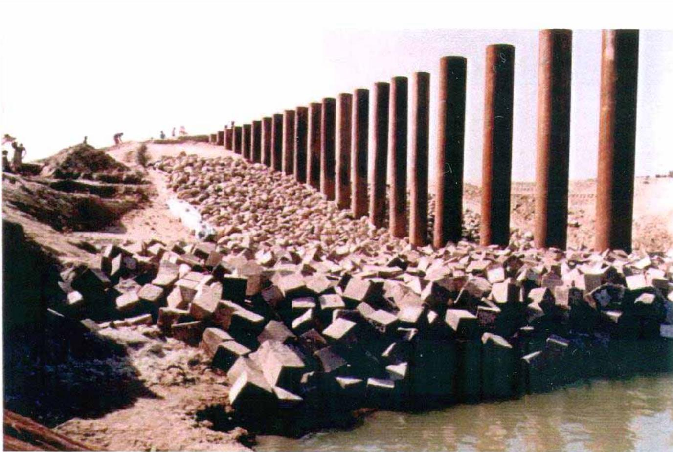
**Photo 7.9-5: Groyne G-2, Bed Protection, dumped CC-Blocks (without filter layer)**
