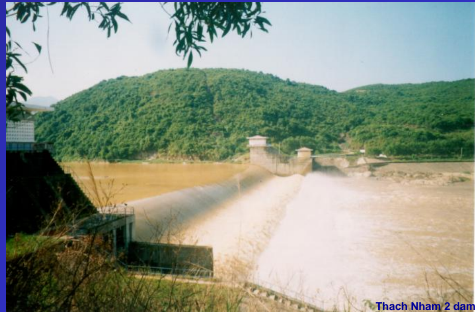
Thach Nham 2 dam
