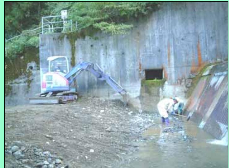
Removal of Rock and Sand
