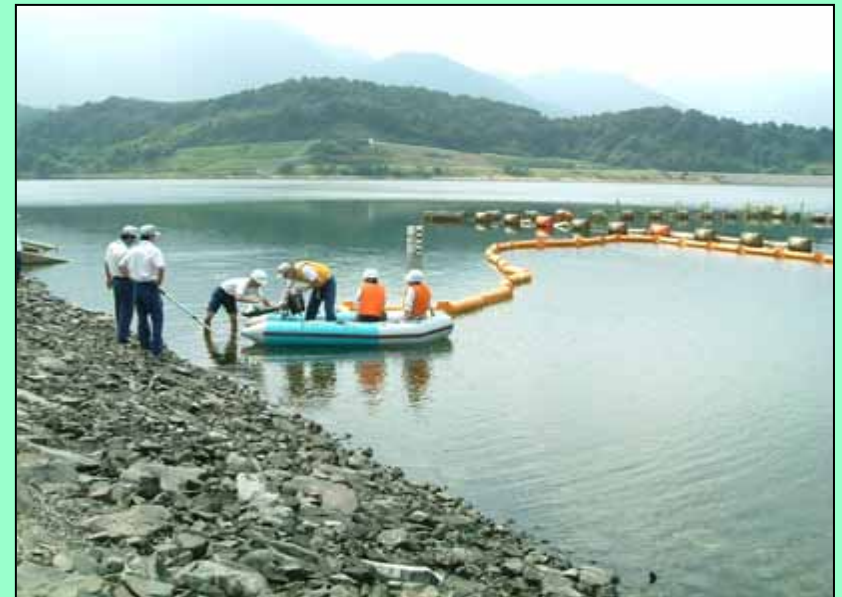
Measures for water pollution
