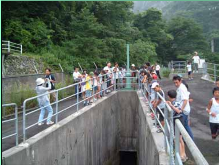
INABE Intake Works
