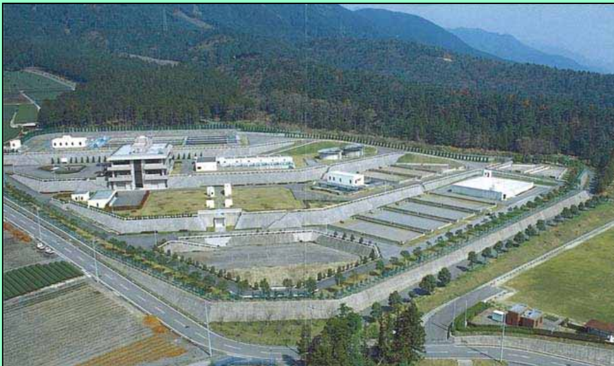
SUIZAWA Water Purification Plant
