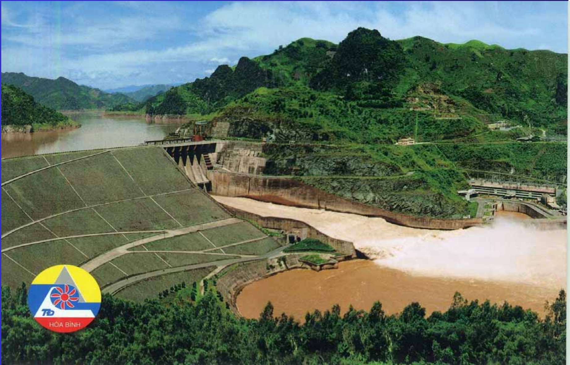
Hoa Binh Hydropower plant
