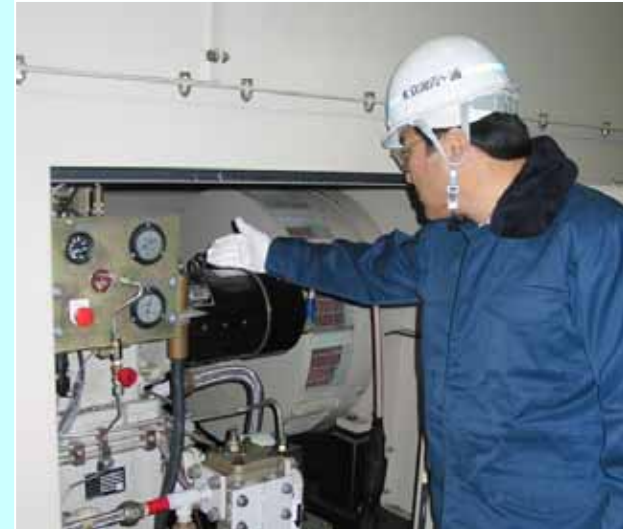
Emergency Generator Equipment inspection
