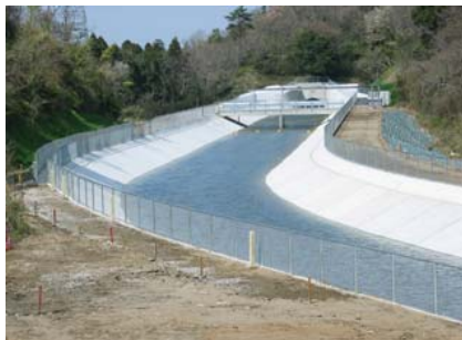
Northern Main Canal
