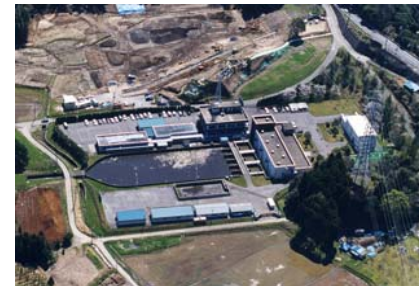
Yokoshiba Pumping Station
