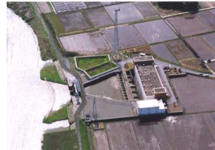
Yokoshiba Pumping Station
