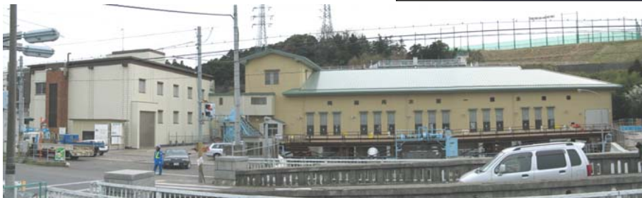
No.1 Ryoso Pumping Station
