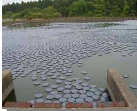
▲Hexagon floats used for restraint of algae or water bloom
