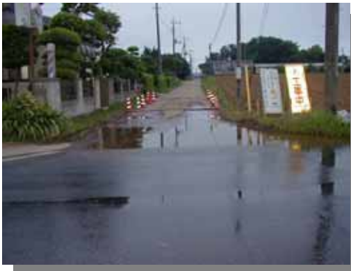
▲Flooded local street due to water leakage
