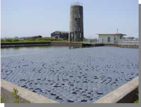
▲Shinden farm pond as part of Toso Canal facilities
