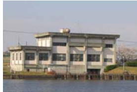
Sogo Irrigation and Drainage Pumping Station to be improved
