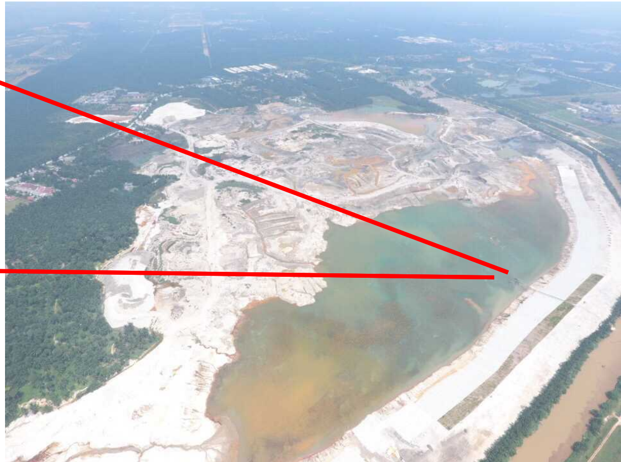
4. HORAS 600 Pond - 8 pumps by KSSB
