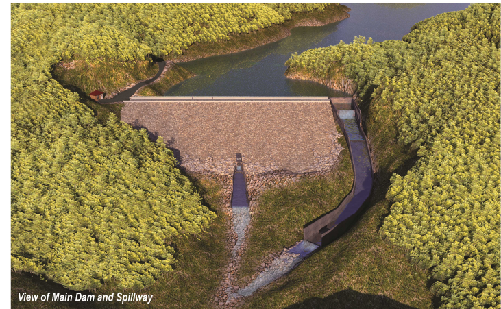
View of Main Dam and Spillway
