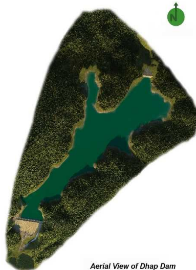
Aerial View of Dhap Dam
