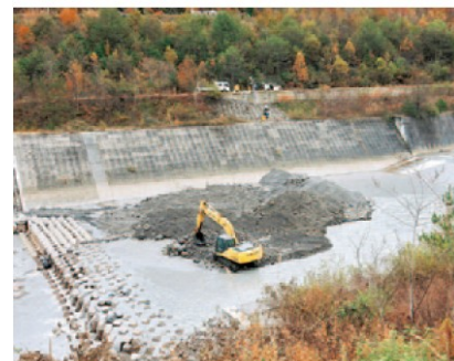
Removal of volcanic ashes from Mt. Ontake (Makio Dam-Aichi Canal)
