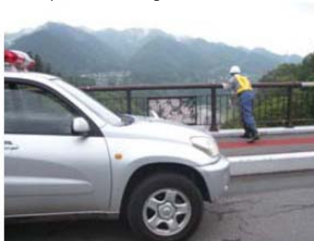
Facility patrol by car at the Takizawa Dam
