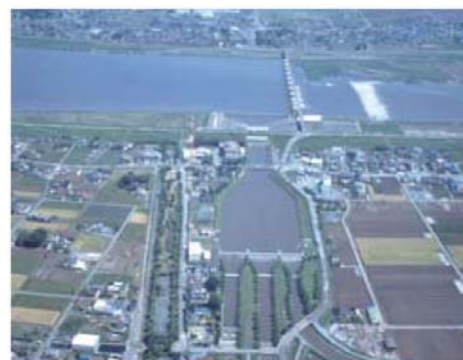
Taking water from the Tone River to Gunma, Saitama, and Tokyo prefectures at the Tone Large Barrage
