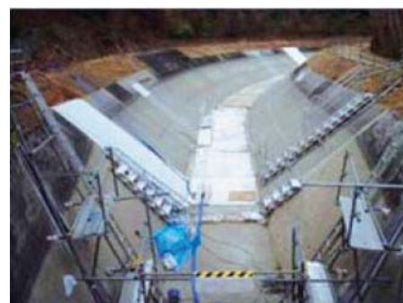
Partial replacement of the lining
