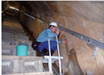
Measuring the leakage inside the body (Shimokubo Dam)
