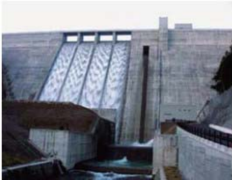
Oyama Dam construction project (completed in FY2012)
