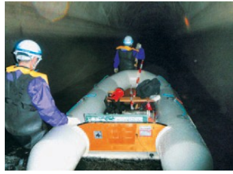
Inspecting the inside of a tunnel (Kasumigaura Canal)
