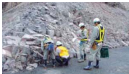
Supervision of work to construct the dam body
