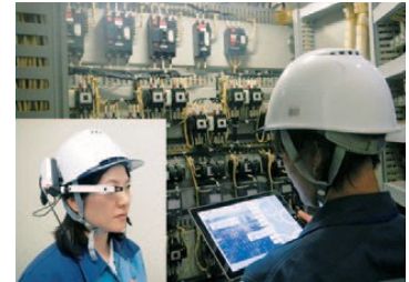
Facility operation support, using a head-mounted tablet display (Trial run) (Lake Biwa Development)
