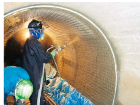
Ryochiku-heiya Canal Stage II (Reinforcement of inner tunnel surface)
