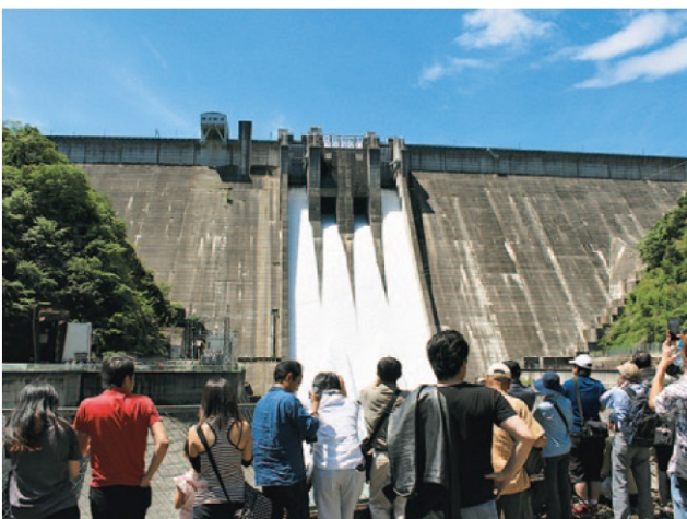
Gate inspection discharge-opening to the public (Shimokubo Dam)
