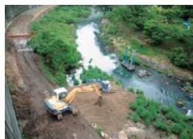
In 2003, gravel and sand were thrown in with a heavy machine
