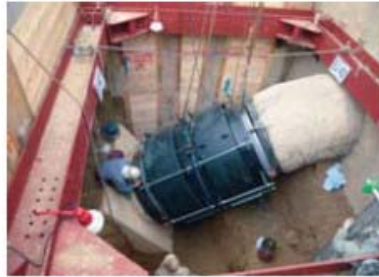
Aseismic engineering (replacing a flexible pipe) (Fukuoka Headrace)
