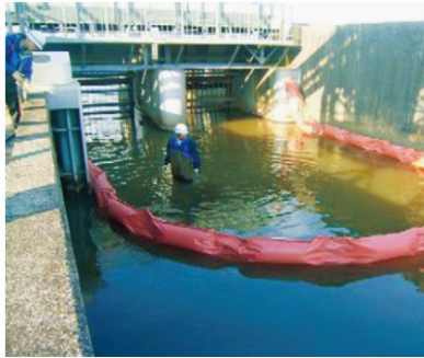
An oil fence is installed across the Kisogawa Canal to address a water quality hazard
