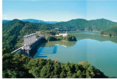
Rain fills the the Sameura Dam Reservoir September 5, 2013 (storage rate: 100%)
