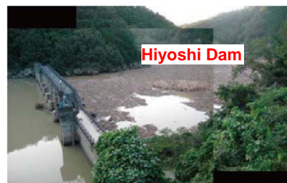
The Hiyoshi Dam blocks driftwood.
