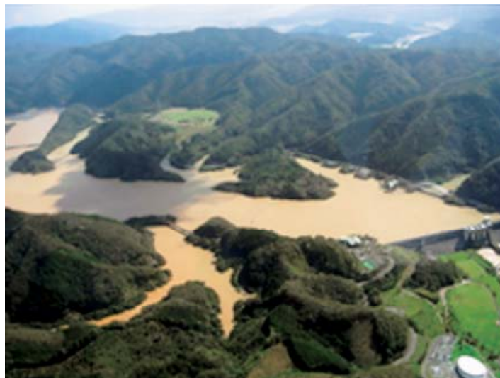
Hiyoshi Dam having stored maximum water (Picture taken by Kinki Regional Development Bureau, MLIT)
