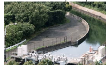
Futagawa Power Station (Toyogawa Canal)
