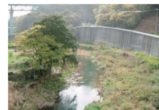
In 2002, about 20 years passed since management start. The river condition was bad. Gravel and sand are gone and grasses and bushes were growing.
