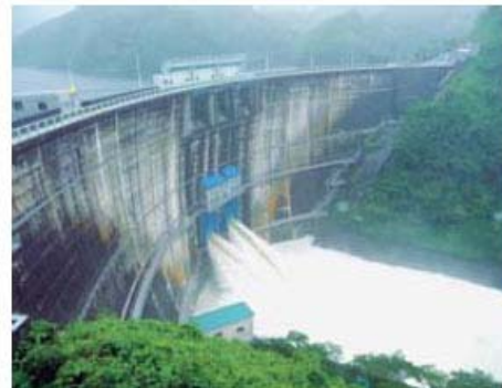
Flood control at the Shorenji Dam
