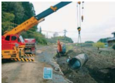
Replacing a branch pipeline at the Kisogawa Canal
