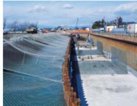
Musashi Canal reconstruction project (Change to double-way canal)
