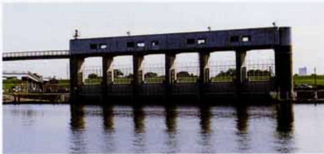
Front View of Muneoka Intake Gate
