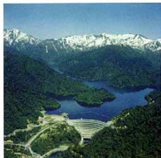
Yagisawa Dam (Tone River System)
