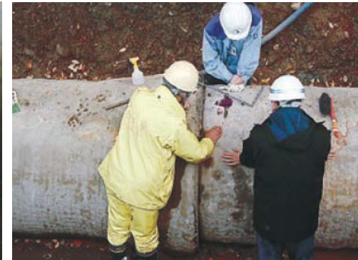
Inspection of aging status of pre-stressed concrete pipe
