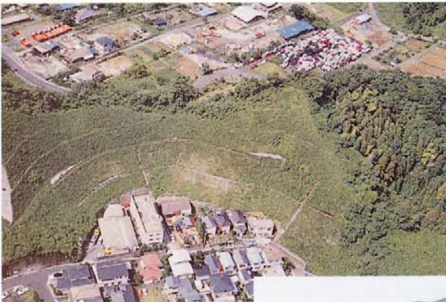
Several years after the building of prevention works
