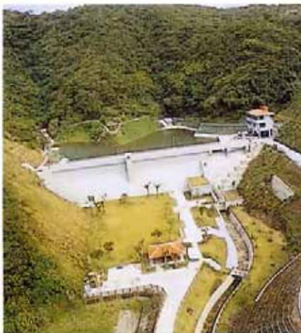
Zamami Dam (Okinawa prefecture)
