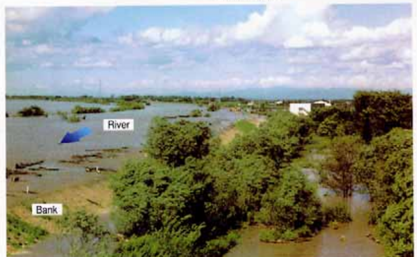
Trees reduce the energy of overbank flow and project the levees.
