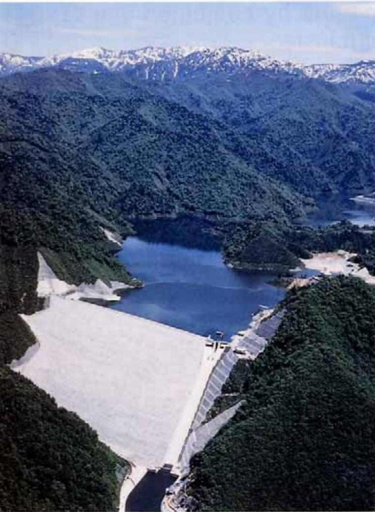
Naramata Dam (Gunma pref.)
