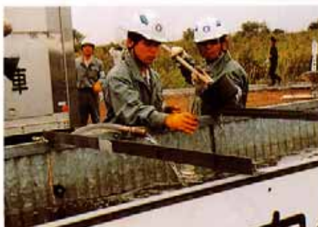
Contaminated water is collected and treated with oil collectors and oil separators, and treated water is returned to the river.
