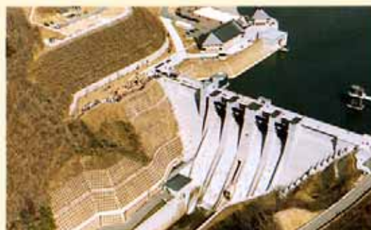
Dam designed to well with surrounding landscape (Miharu Dam, Tohoku Regional Development Bureau)
