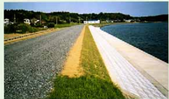
Lake shore levee (Lake Kasumigaura Development, Water Resources Development Public Corporation)
