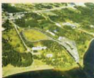
Man-made section of the Ado River
