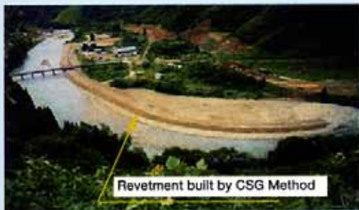
Full view of completed revetment
