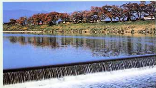
Keeping running water clean
