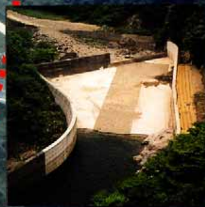
Improvement and construction of energy dissipator
