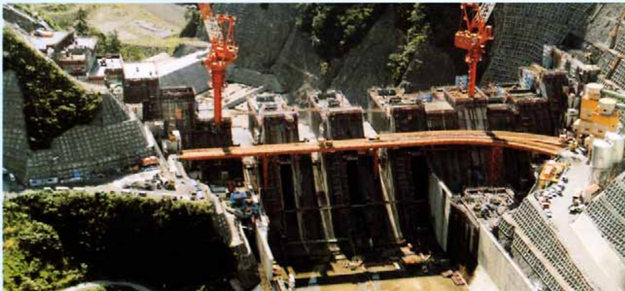
Nagashima Dam (Chubu Regional Development Bureau)
