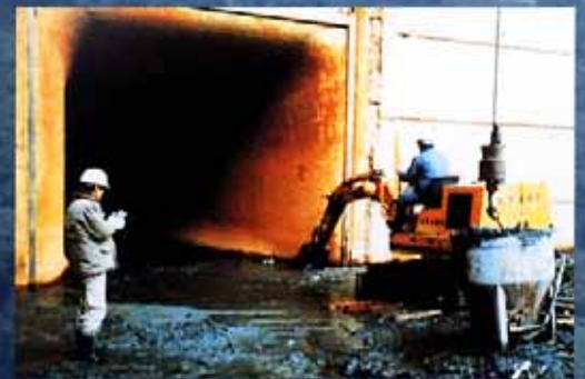
Improvement or construction of spillways, gates and other facilities
