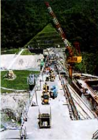
Satunagawa Dam (Hokkaido Development Bureau)
