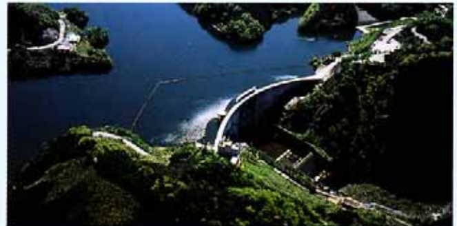
Shorenji Dam (Water Resources Development Public Corporation)
