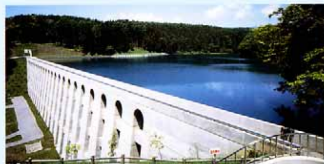
Sasanagare Dam (Hakodate City)
