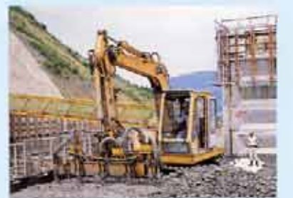
Crawler-mounted vibrator used for compaction
