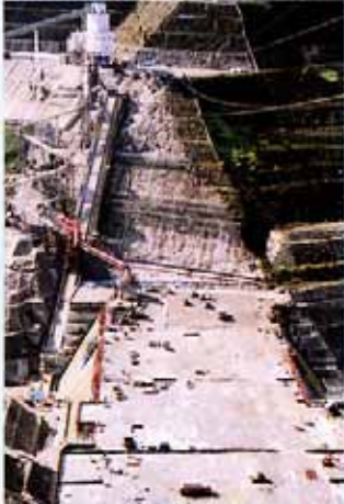
Gassan Dam (Tohoku Regional Development Bureau)
