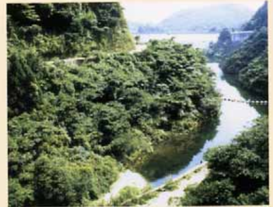
Lakeside slope 10 years after completion of the dam (1993)
