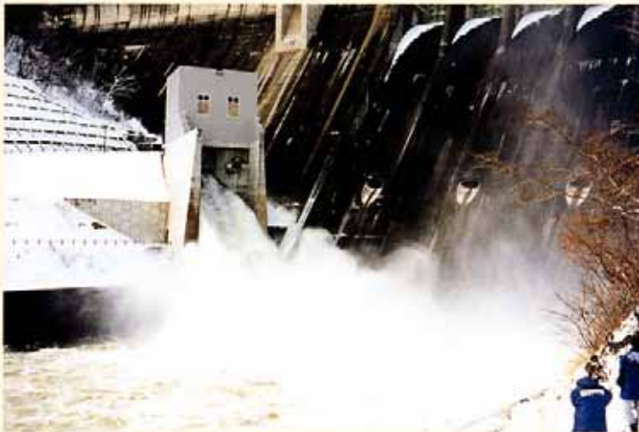
Tase Dam (Tohoku Regional Development Bureau)
