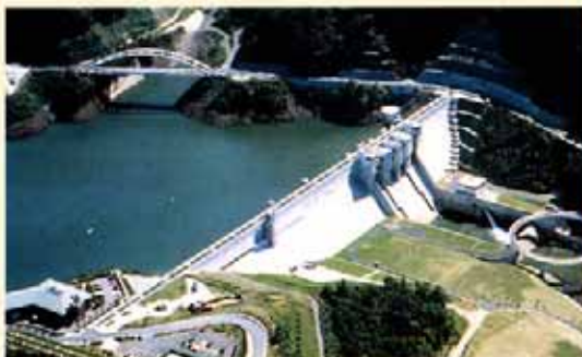
Dam body and plaza opened to the public for upstream-downstream exchanges (Hiyoshi Dam, Water Resources Development Public Corporation)
