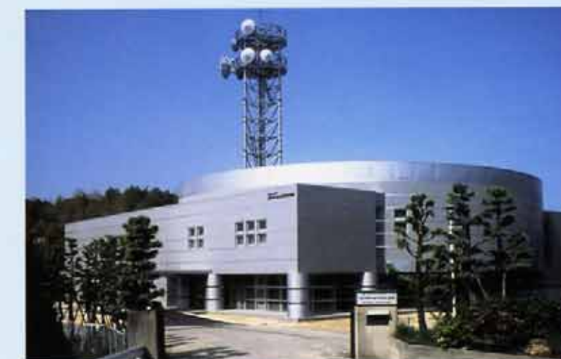
Yodogawa dam Integrated Control Office
