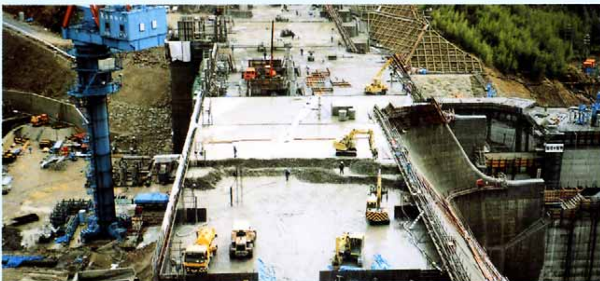
Hinati Dam (Water Resources Development Public Corporation)
