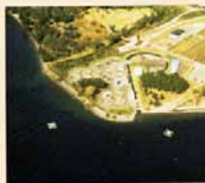
Man-made section of the Ane River
