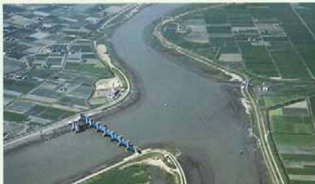
Providing a secure water supply for existing irrigation uses
