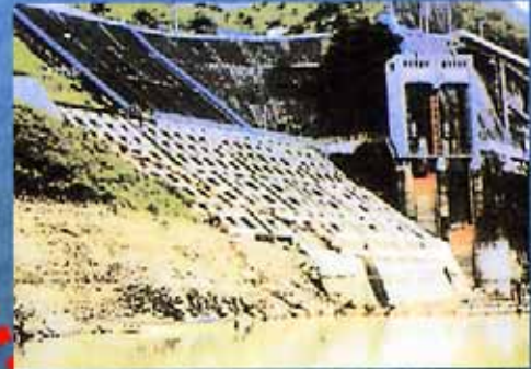
Extensive slope stabilization works around dam body
