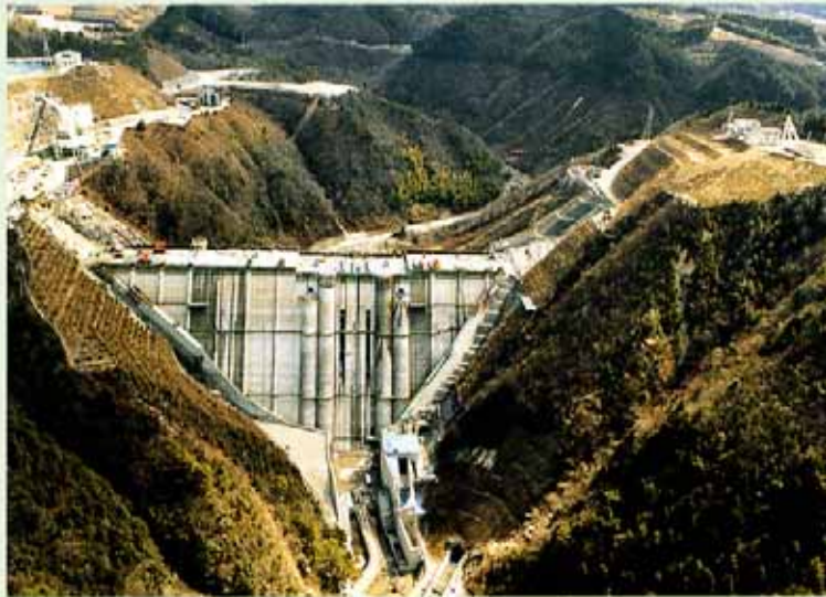
Origawa Dam (Chubu Regional Construction Bureau)
