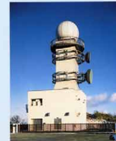
Radar rain gauge station
