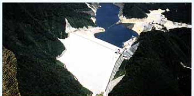
Naramata Dam (Water Resources Development Public Corporation)
