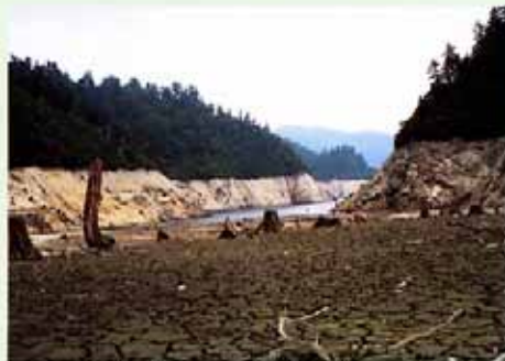
Reservoir bottom exposed during drought (Drought of 1990, Yagisawa Dam)
