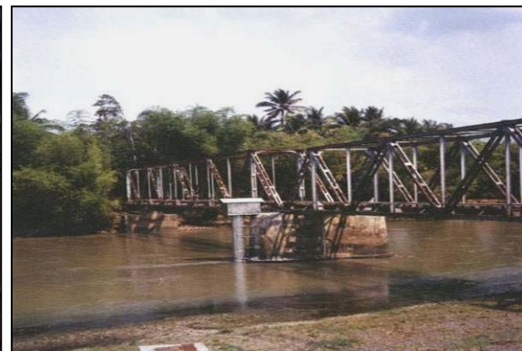
Water level gauging station
