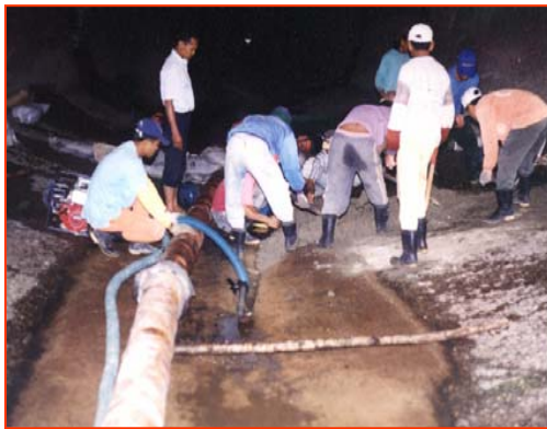
REHABILITATION OF TUNNEL
