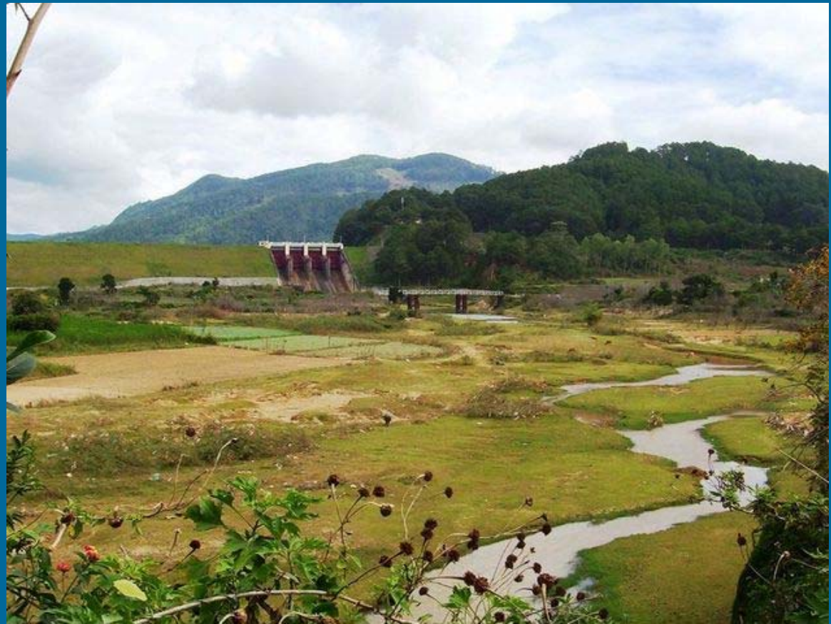
Da Nhim hydropower in the dry season
