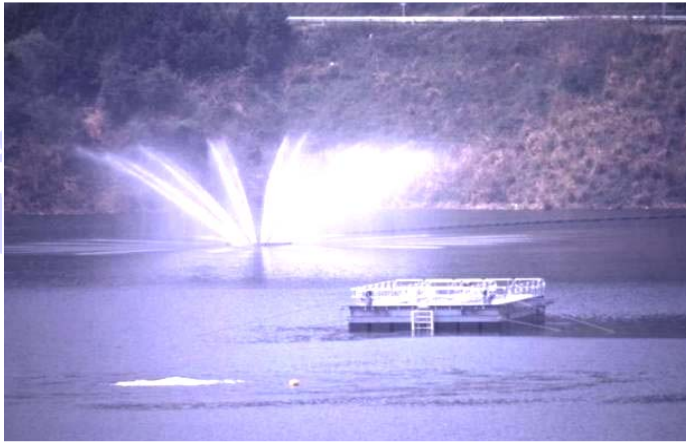
Hypolimnion Aeration (front) and Surface Aeration (back)
