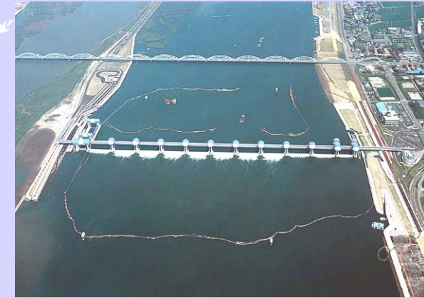
Nagaragawa Estuary Barrage
