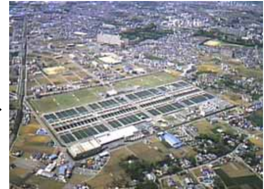
Asagiri water purification plant (Tokyo)
