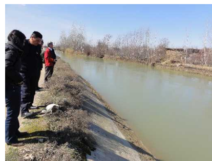
Uzbekistan North Fergana canal
