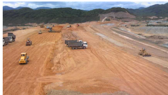
Photo: Dam Construction (9million cubic m)
