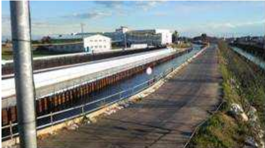
Photo: Re-construction of the aged canal using the elaborate technology
