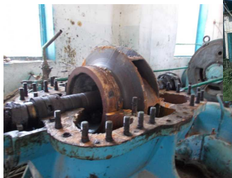
Malfunctioned water pump and motor
