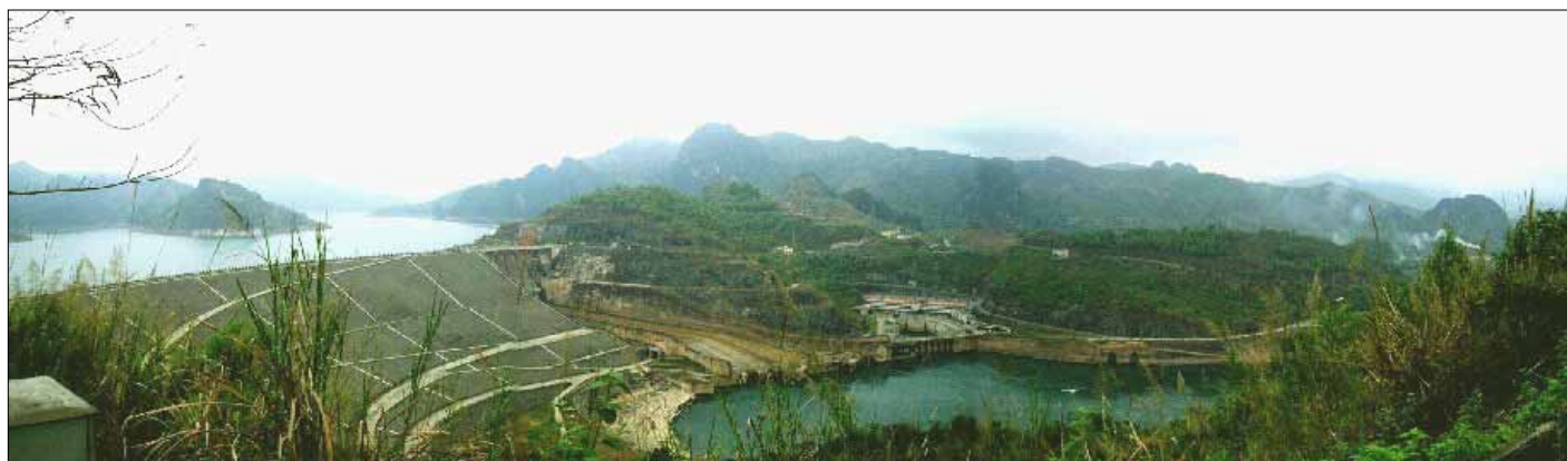
Hoa Binh reservoir, one of the most important water infrastructures in the Red – Thai Binh river basin
