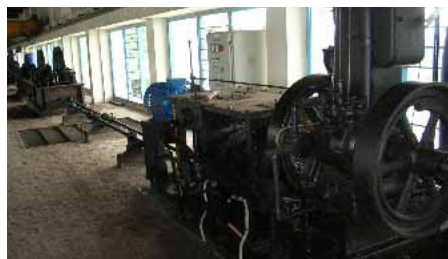
Steam engine which move gate up and down for more than 80 years
