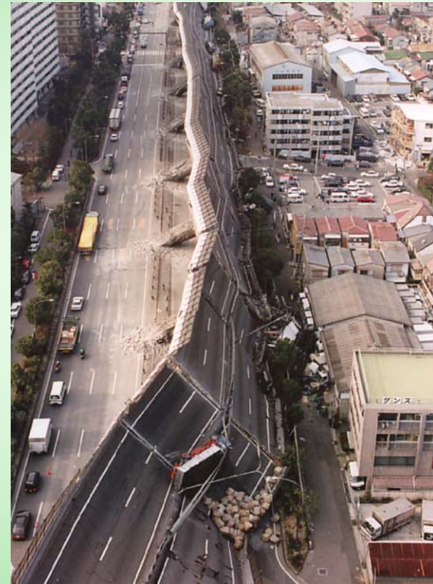
Collapse of an expressway after the Hanshin Awaji Earthquake
