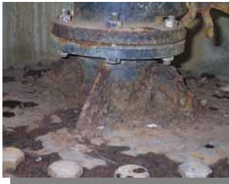
▲Degraded part of air valve
