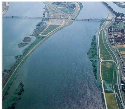
The mound section after dredging (photographed in September 2000)
