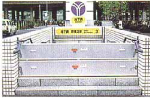
Figure 5.6 Installation of Flood Control Device (Water Barrier Boards)
