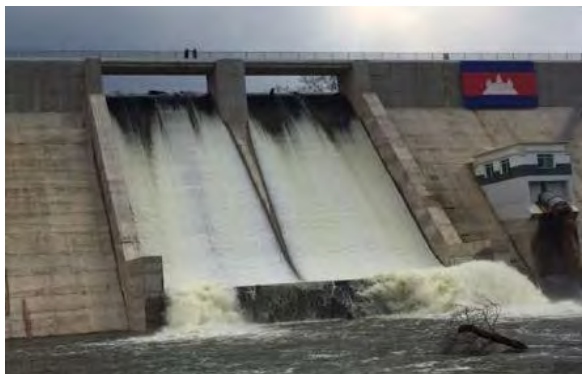
Barrage for diversion water to irrigation system
