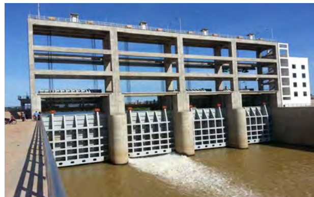
Barrage for diversion water to irrigation system
