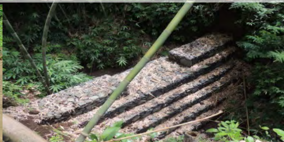
Check dam construction
