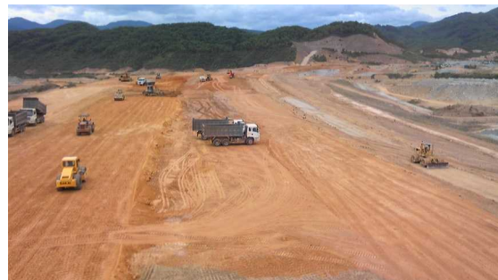
Photo: Dam Construction (9million cubic m)
